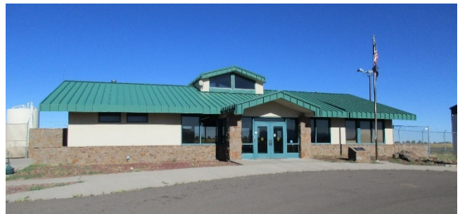
Airport Terminal Building
