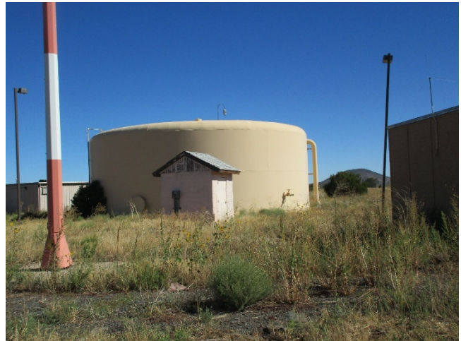
Water Storage Tank and Pumphouse
