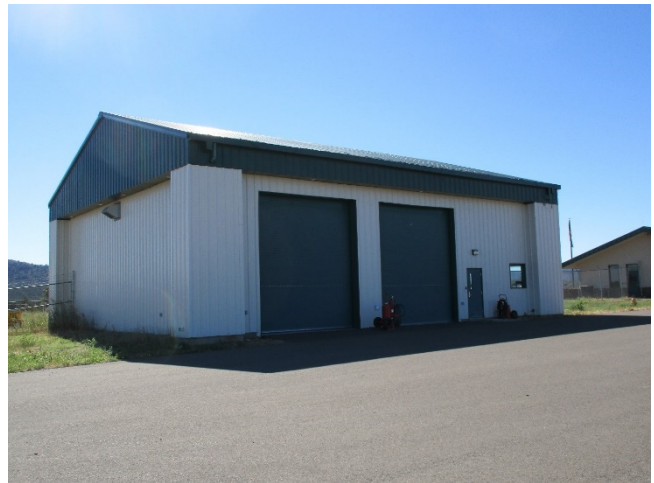
Airport Maintenance/Firefighting Equipment Building
