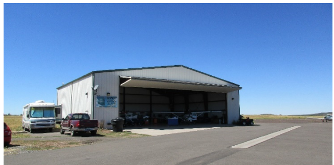
NAZA Maintenance Hangar
