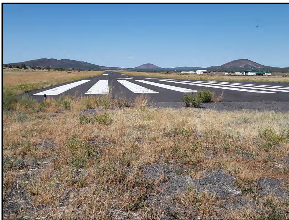
Figure 3. Overview of project area, facing north.
